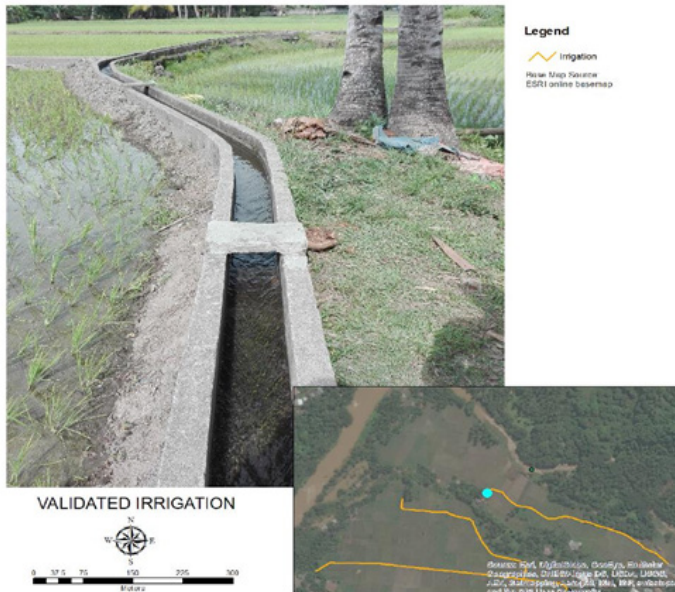
Figure 9. Irrigation Point of Interest in Aerial View and Validated Irrigation in the Ground
